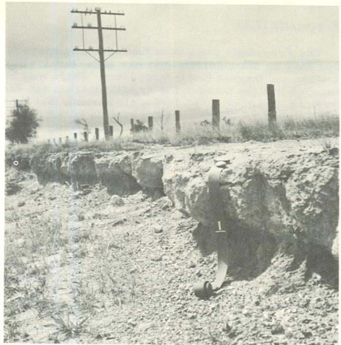
Figure 36.—The hard massive A horizons of Ustalfs often form overhanging shelves in road cuts.
